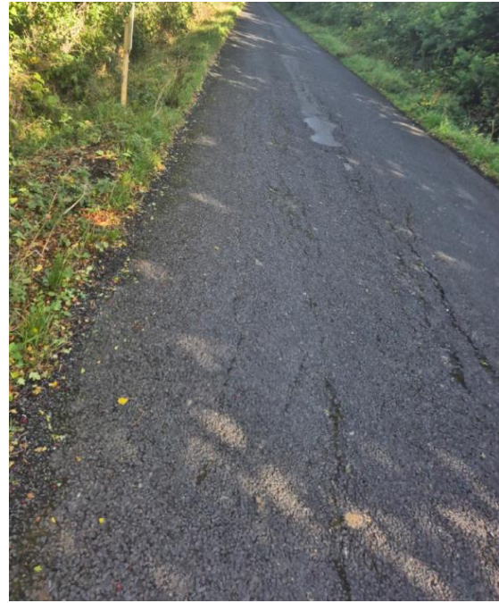
Figure 9 - Adjacent open drain
