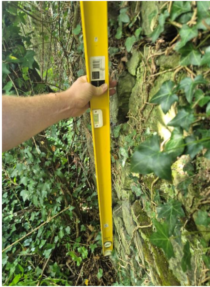
Figure 16 - Bulging of northeastern spandrel wall panel
