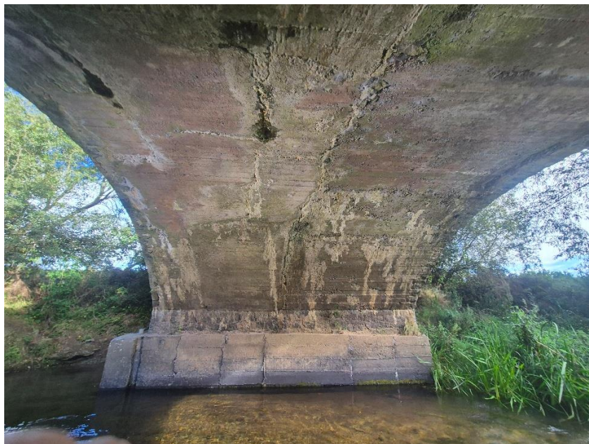
Figure 17 - Central Arch (facing North)
