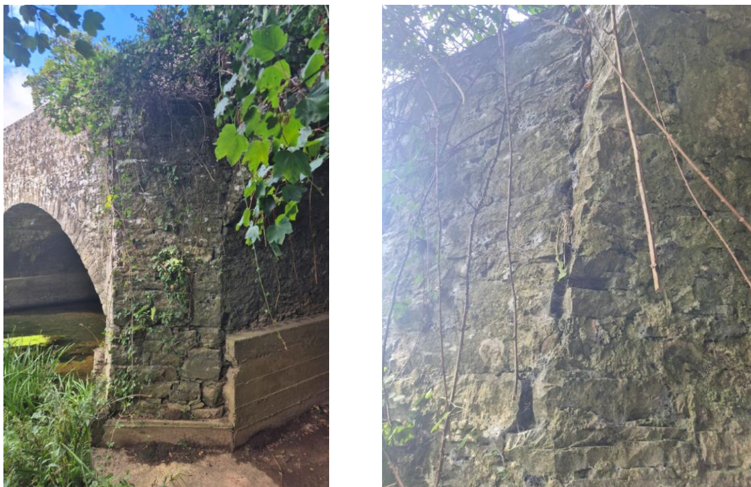
Figure 13 - North/Central arch cutwater
