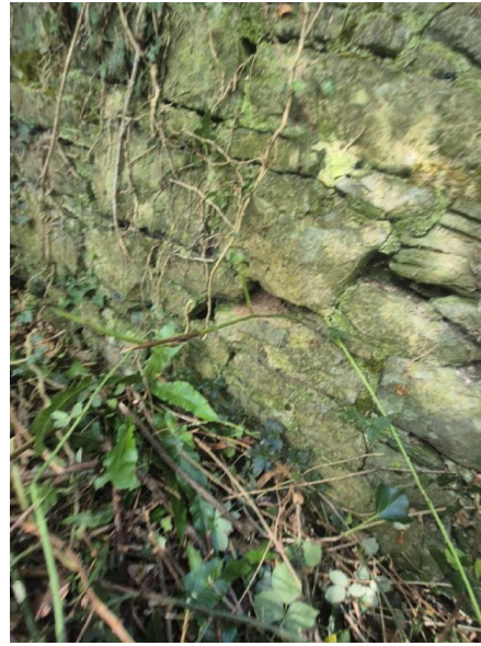
Figure 16 - Bulging of northeastern spandrel wall panel
