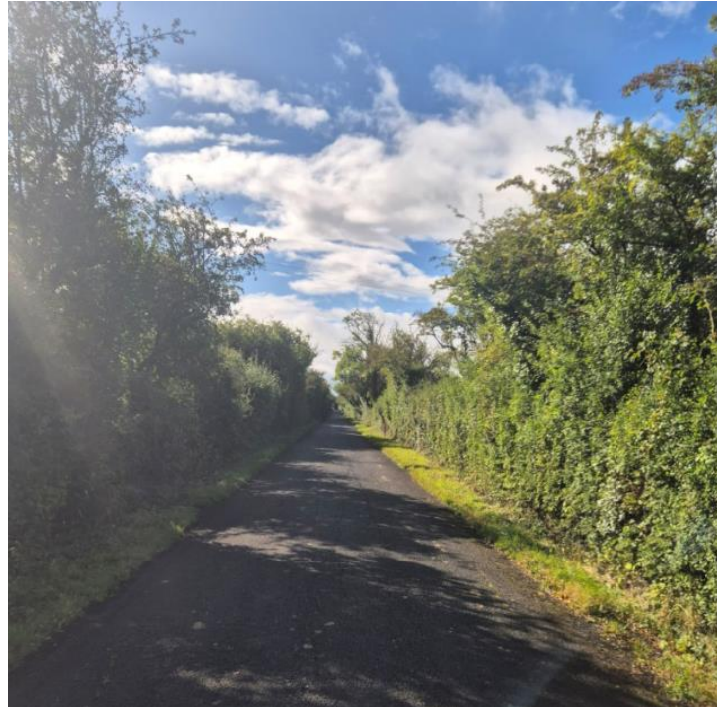
Figure 7 - Southern approach to Garrouse Bridge
