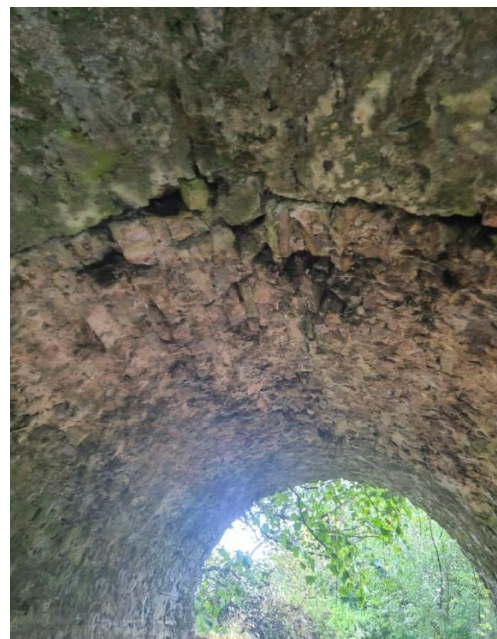
Figure 11 - Crown of Northern Arch
